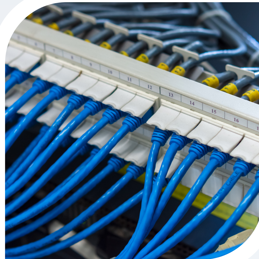
UTP Cable Installation
